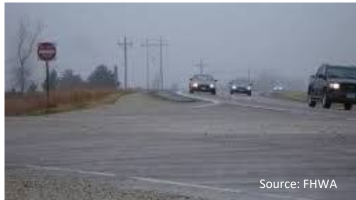
Figure 8. Curve Cross Slope Road Example
