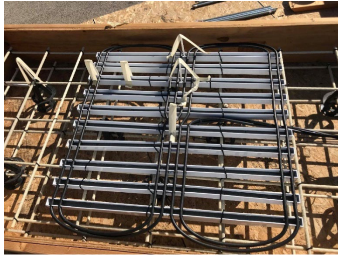
Figure 3.12 PVC tubes installed on IPTs system
