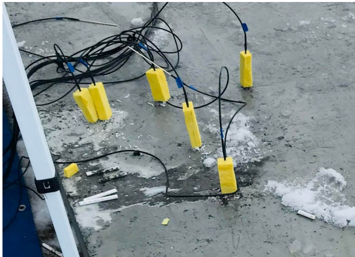
Figure 3.15 Temperature sensors, covered by insulation, inserted into the tubes
