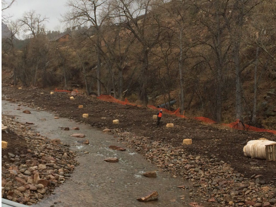
Figure 3.2 Remediation efforts in the Saint Vrain River following wildfire damage, November 21, 2017. Bales of hay and other natural fibrous materials are being used as reinforcement along the riverbank.
