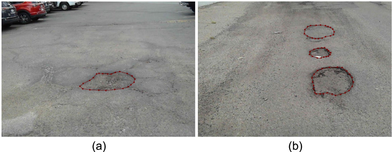
Figure 4.5 Visible images annotation using LabelMe, (a) single pothole, (b) multi-potholes
