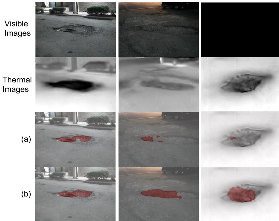
Figure 5.4 Sample results in nighttime for RTFNet, shown for the EP=1.2. (a) EP=1.2 in the first layer, (b) EP=1.2 in all layers
