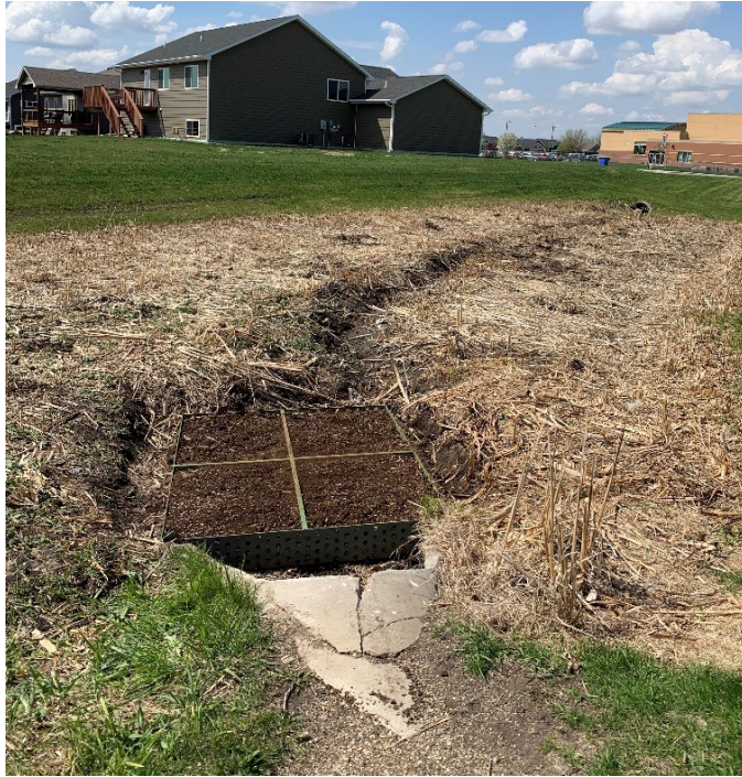
Figure 2.5 Field stormwater filter site location
