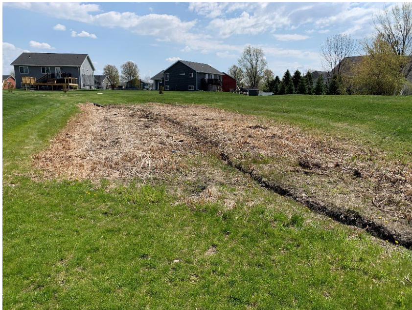
Figure 2.6 Stormwater detention pond for the stormwater filtration study
