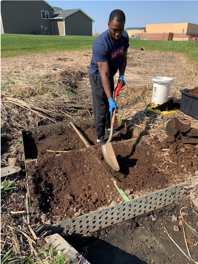
Figure 2.8 Removal of aged materials from the field filter
