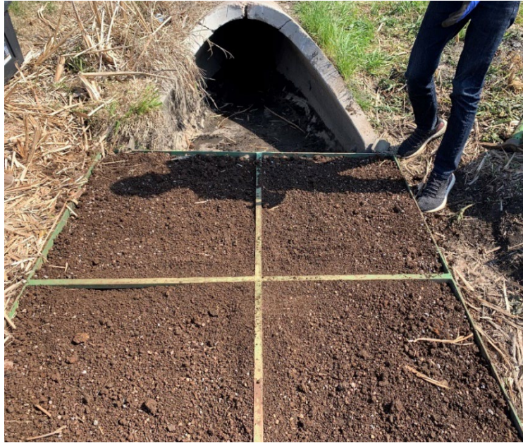
Figure 2.10 Pilot scale steel byproduct filter after ratio adjustment
