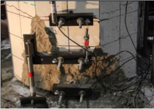
(b) Drift ratio=6% (cracks, spalling, and yield penetration)
