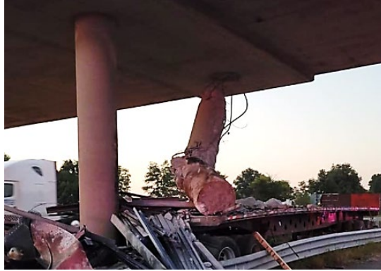
Figure 1.5 Semi-truck collision on the I-55 Bridge, Missouri (2021) [26]
