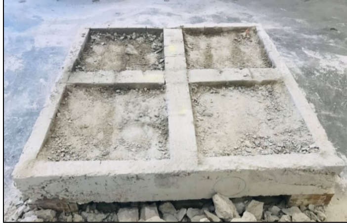
Figure 4.12 The concrete slab after jackhammer removal
