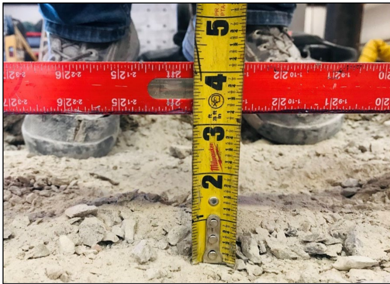
Figure 4.13 Verifying the removal depth
