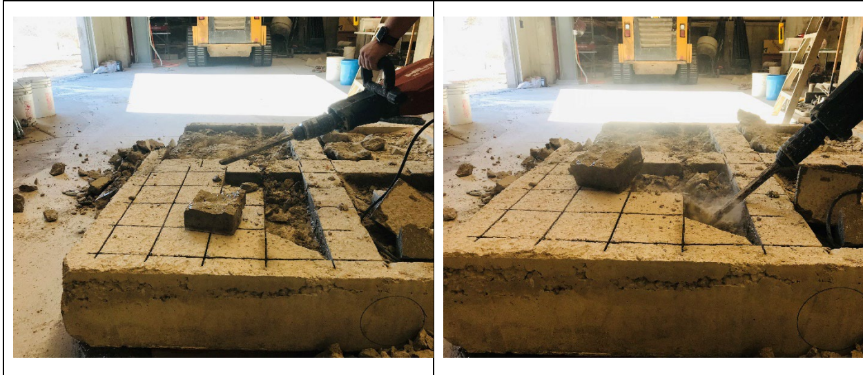
Figure 4.19 Removal of the discretized concrete pieces
