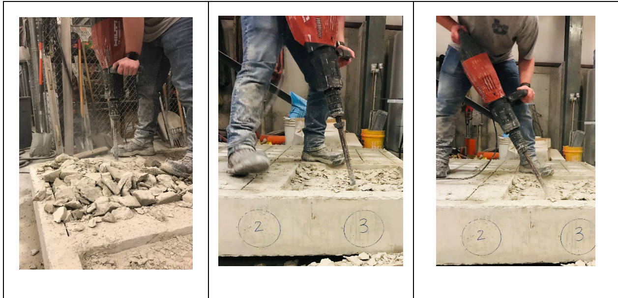
Figure 4.17 Examples of pull-off/impact angles of the jackhammer
