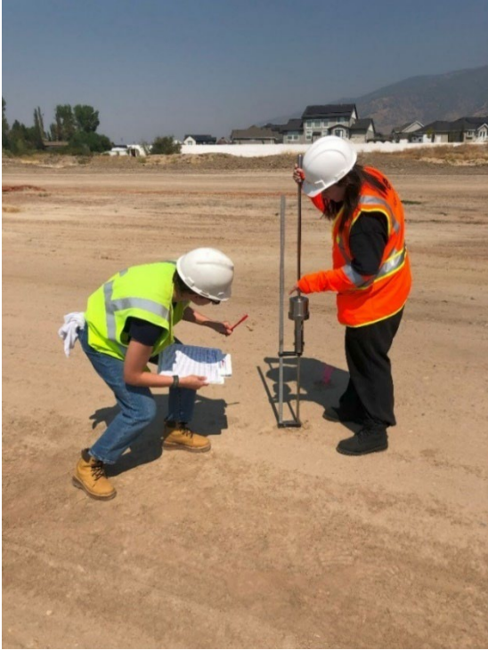
Figure 3.13 Photo of DCP testing being performed on the original subgrade
