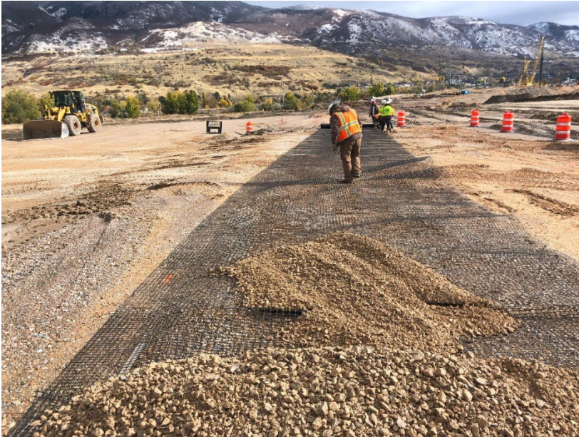
Figure 3.18 Photo showing geogrid being folded during installation
