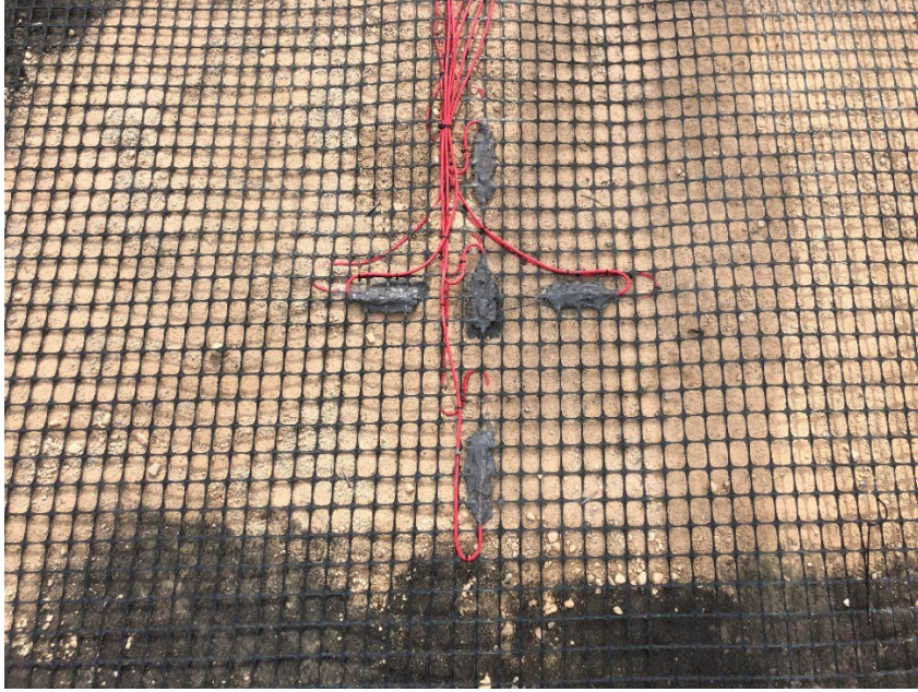
Figure 3.11 Strain gage array installed on geogrid in the field
