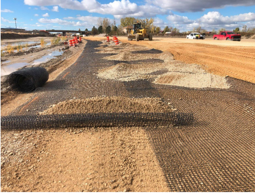
Figure 3.19 Photo showing folds in geogrid during installation
