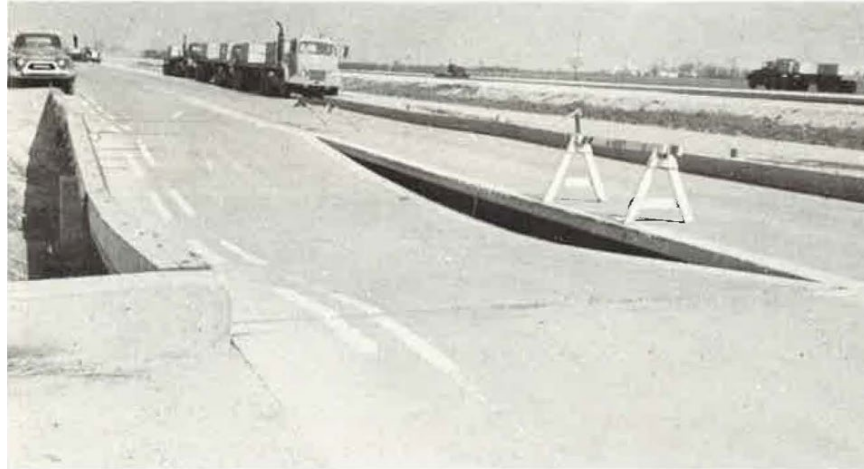
Figure E.2 Bridge testing at AASHO Road Test (10)
