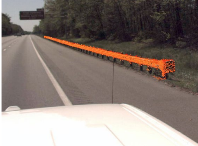
Figure 2.7 An Example of Guardrail Scan And Automatic Extraction by Pillar
