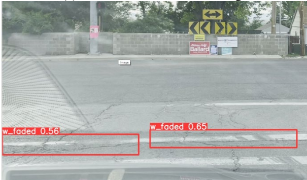
(e) Faded white stop lane markings
