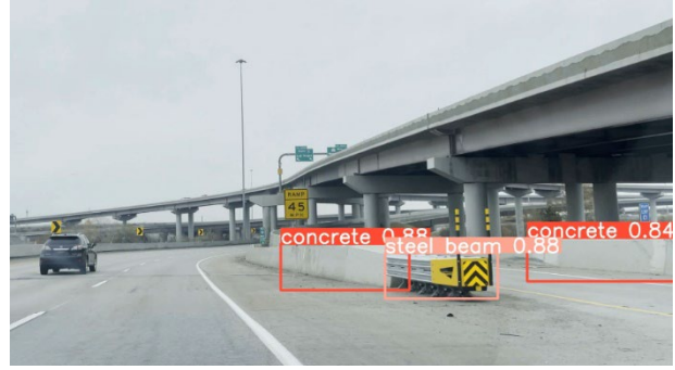
(b) Concrete barrier and steel guardrail
