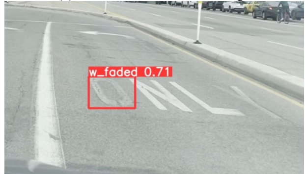
(f) Faded white delineator markings
