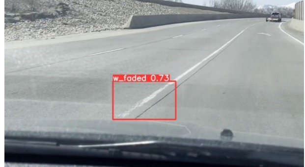
(b) Faded white lane marking
