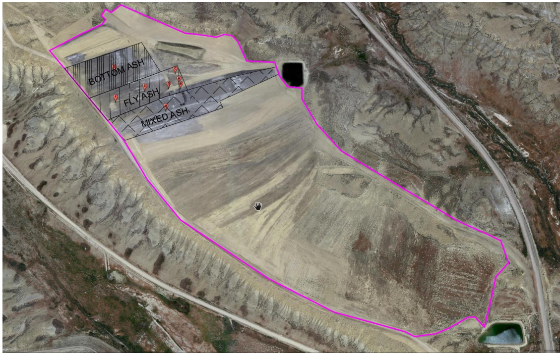
Figure 2.6 Industrial landfill with active cells
