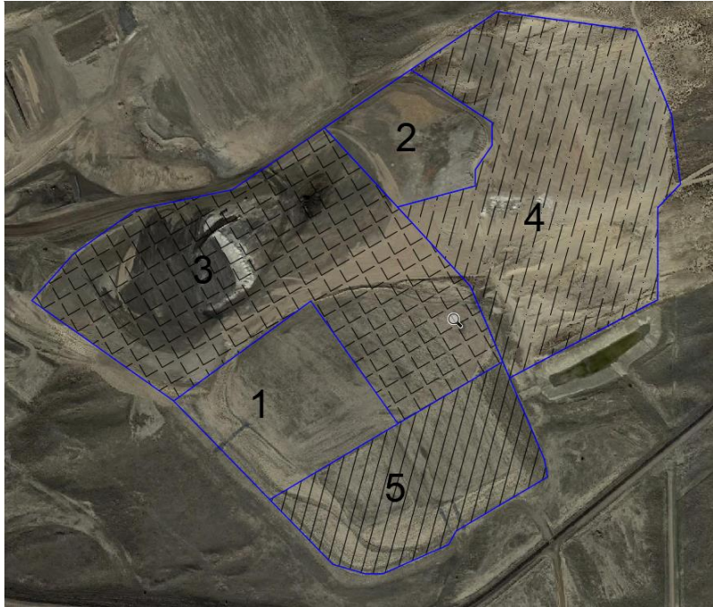
Figure 2.8 Expansion landfill at Dave Johnston Power Plant
