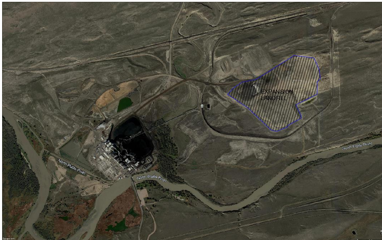
Figure 2.4 Dave Johnston Power Plant with the expansion landfill
