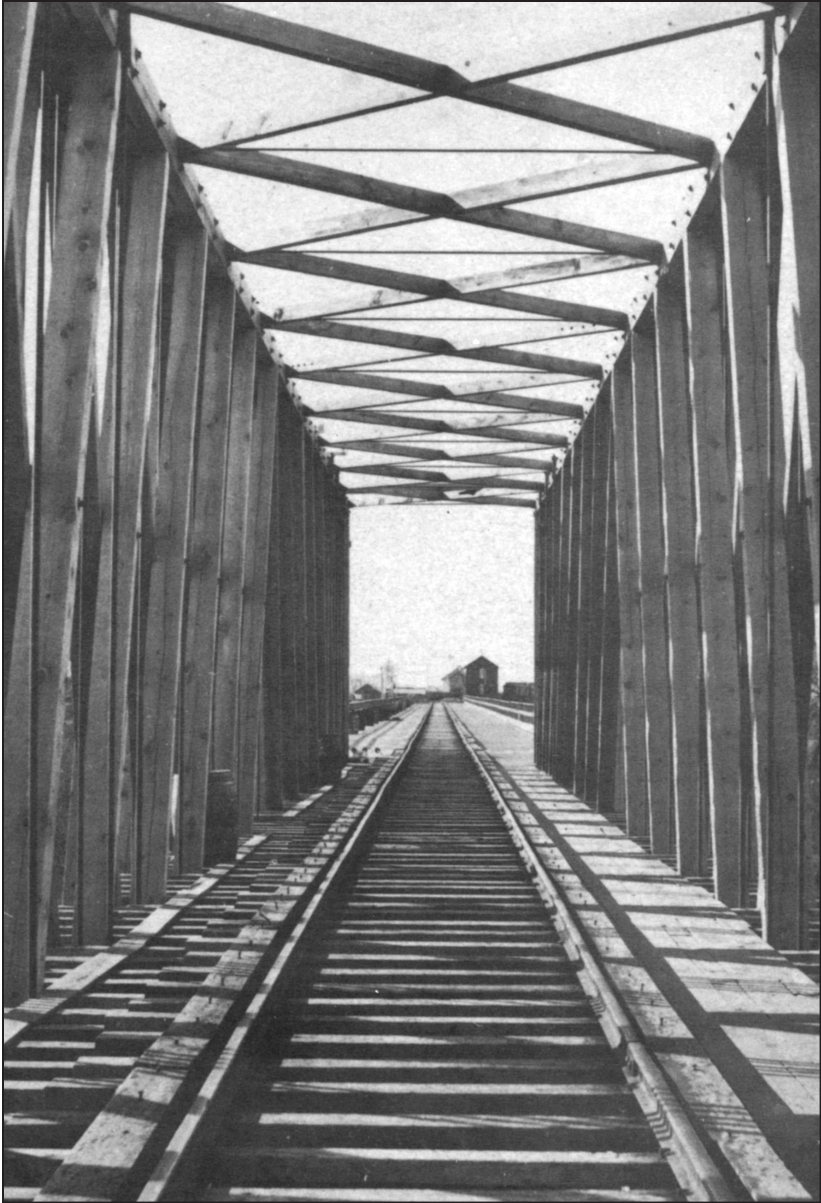
Viewing down the interior of the Northern Pacific bridge from Moorhead
