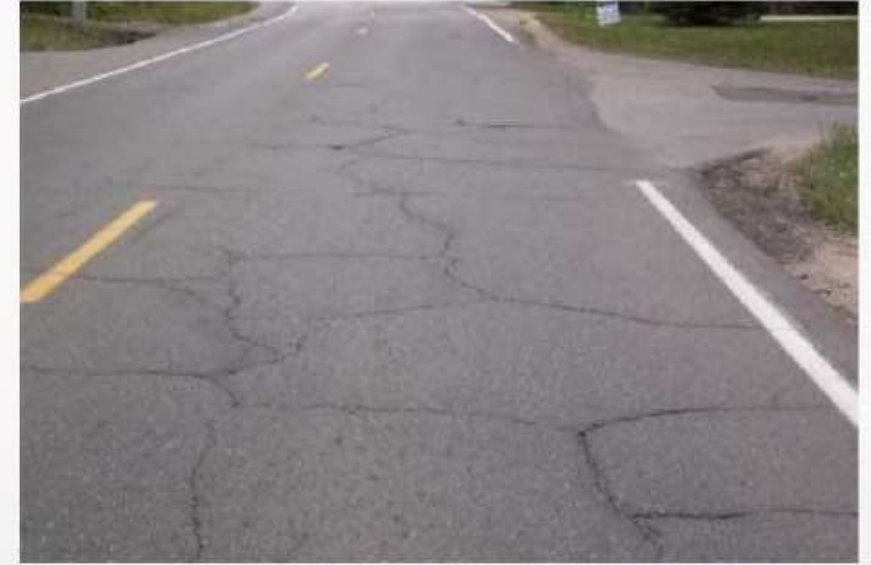
Fatigue Cracking
