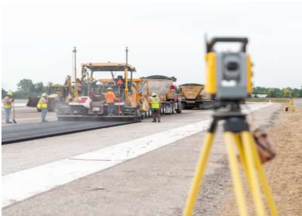
"trimble 3d asphalt paving" | Search | LinkedIn
