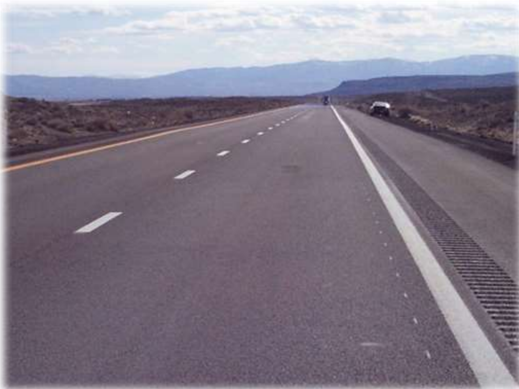
PG 64-22 modified, no rutting
