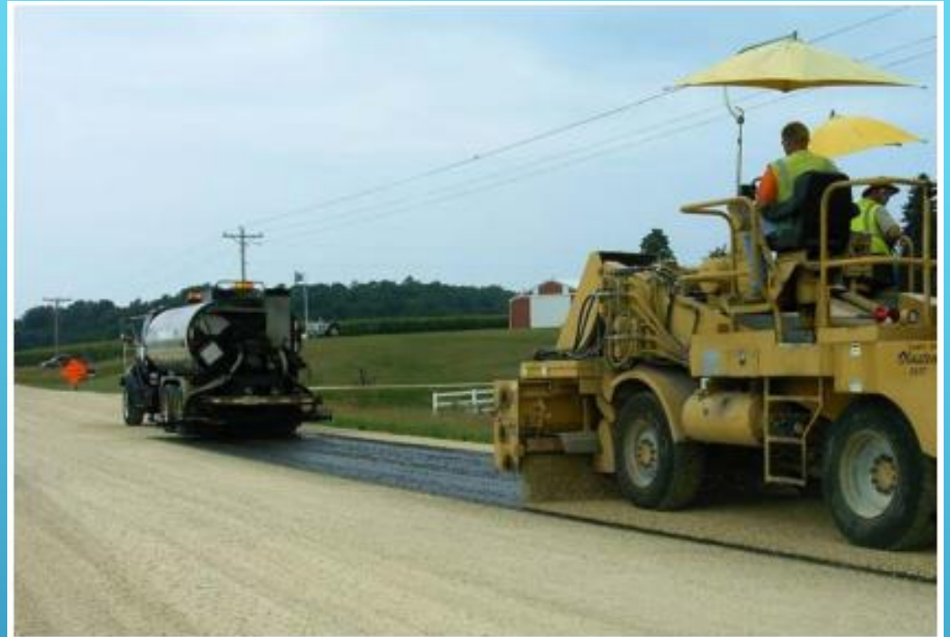
Otta Seal Const. 2007, Olmsted County CR58
