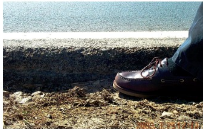
Photo Source: FHWA
