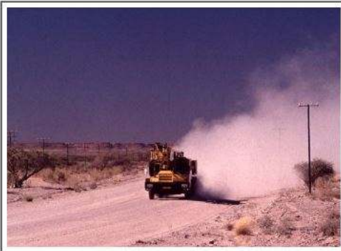
Loss of fines (as dust) on an untreated road
