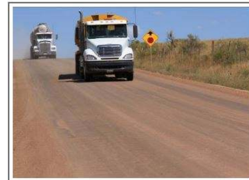
Stable fines preservation on a treated road
