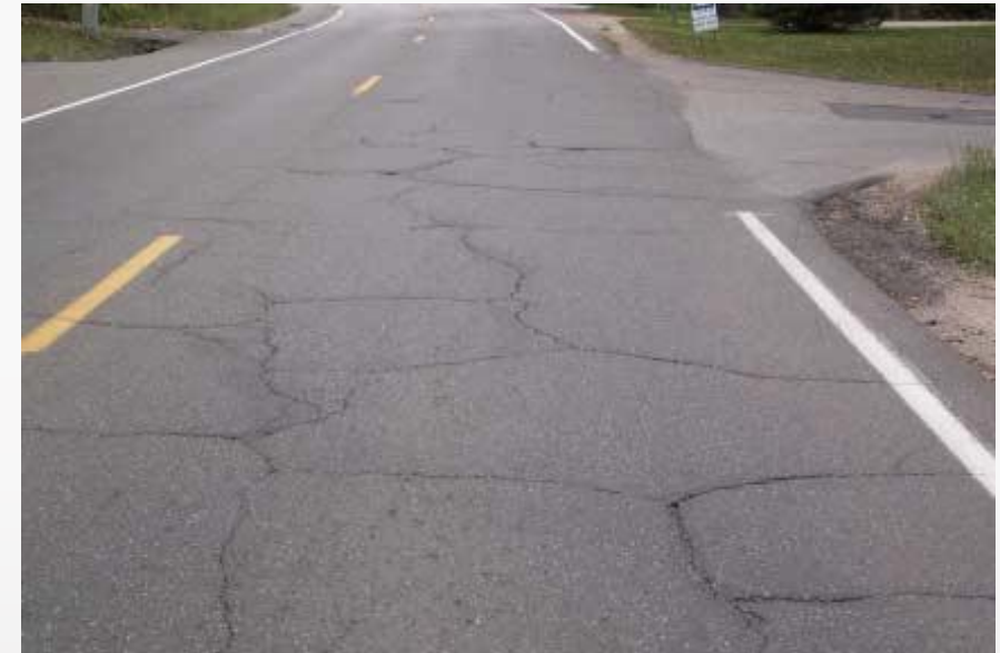
Fatigue Cracking
