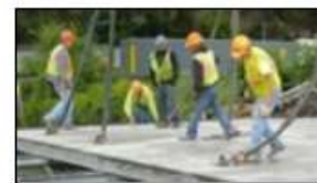
Ultra-High Performance Concrete Connections
