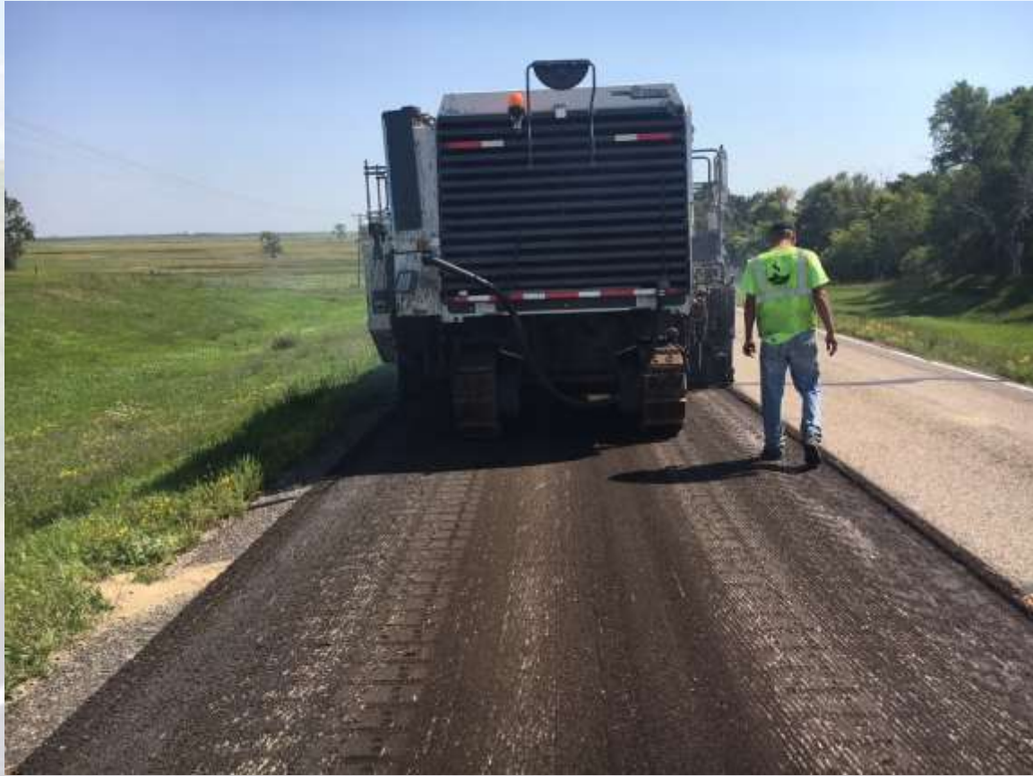
12 foot Micro-Mill – rumble strips are gone
