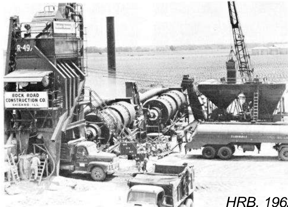
Figure 92. Automatic batch-type plant used to produce binder course mixture; dryers in tandem.
