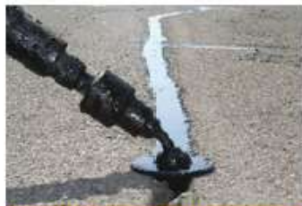
Routed crack being sealed
