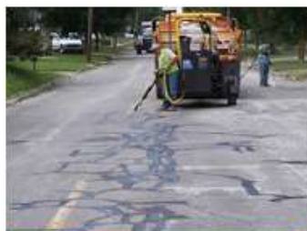
Crack sealing in the field
