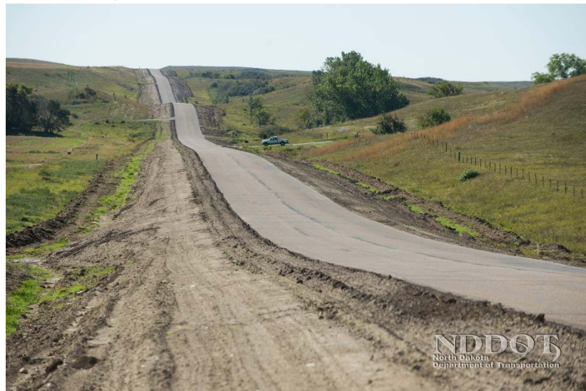
Roadway improvement project in Oliver County.
