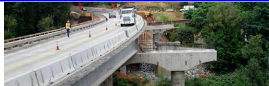
Prefabricated Bridge Elements and Systems
