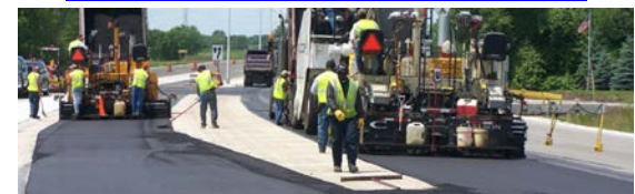
Warm Mix Asphalt
