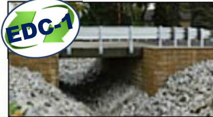
Geosynthetic Reinforced Soil-Integrated Bridge System
