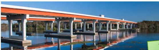
Accelerated Bridge Construction (ABC)
