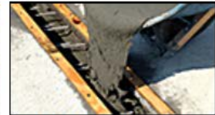
Ultra-High Performance Concrete Connections
