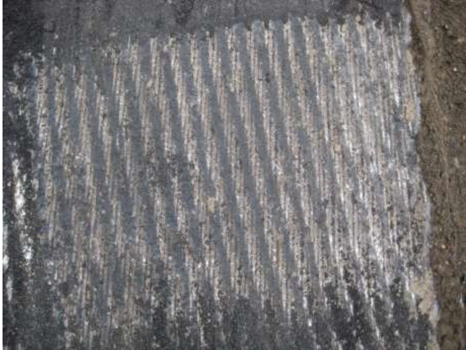
3/8" spaced Single Hit "Profiling" Drum at 120 FPM
